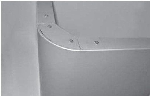
Corner Panel with Gusset and Filler Plate
